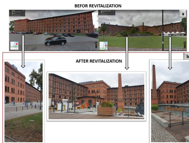
Fig. 5. Rothera Mills: a) view of the building before revitalization – Street View 2017; b) view of the building after revitalization – photographic documentation 2022, by Kinga Szopińska
